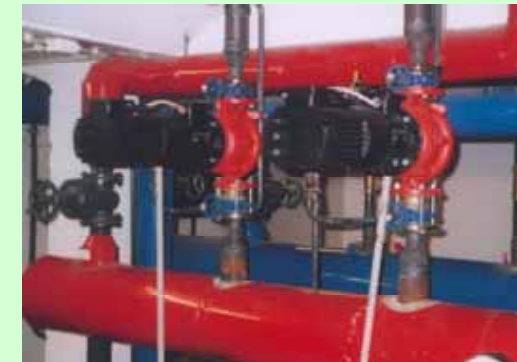
New energy-efficient pumps
