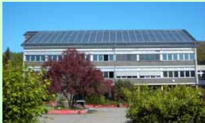
The PV power plant
